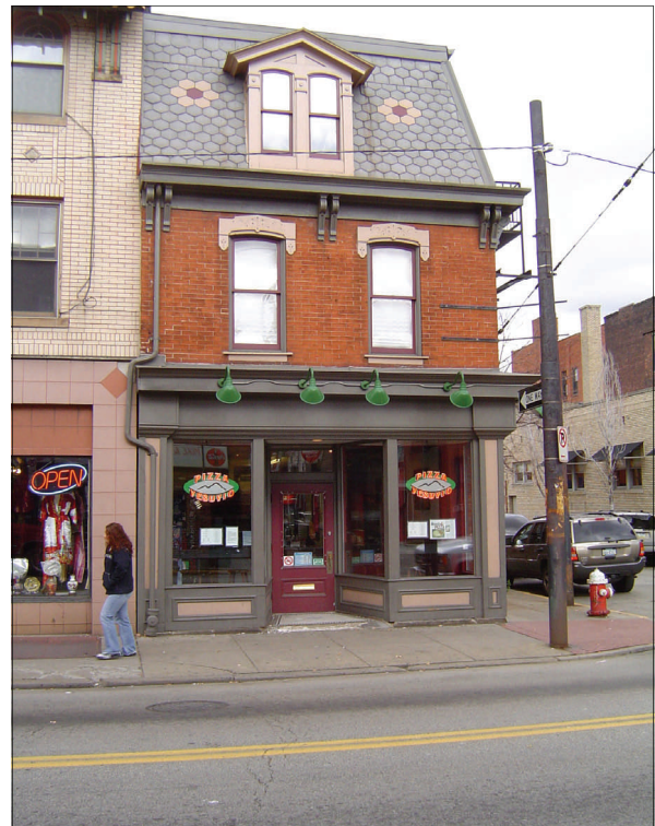
Figure 27. Mansard roof restored with slate
