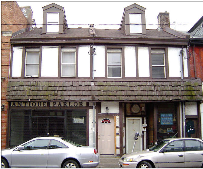
Figure 5. Inappropriate remodeling: inauthentic Tudor details added to a Greek Revival building
