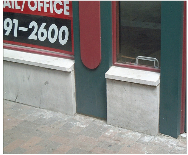
Figure 21. Stone bulkheads below display windows
