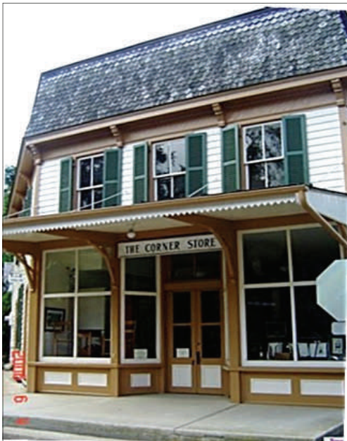
Figure 26. Wood façade restored and painted
