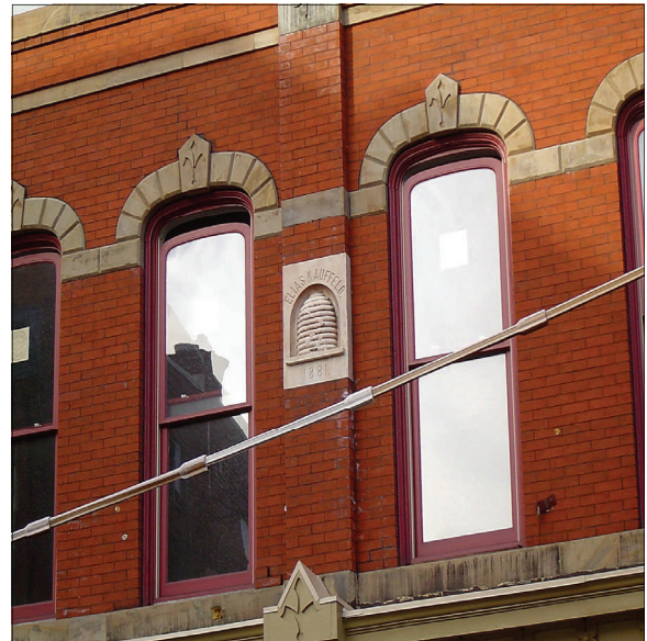
Figure 29. Wood replacement windows with arched tops to fit openings
