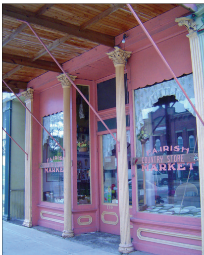
Figure 16. Storefront with recessed entrance
