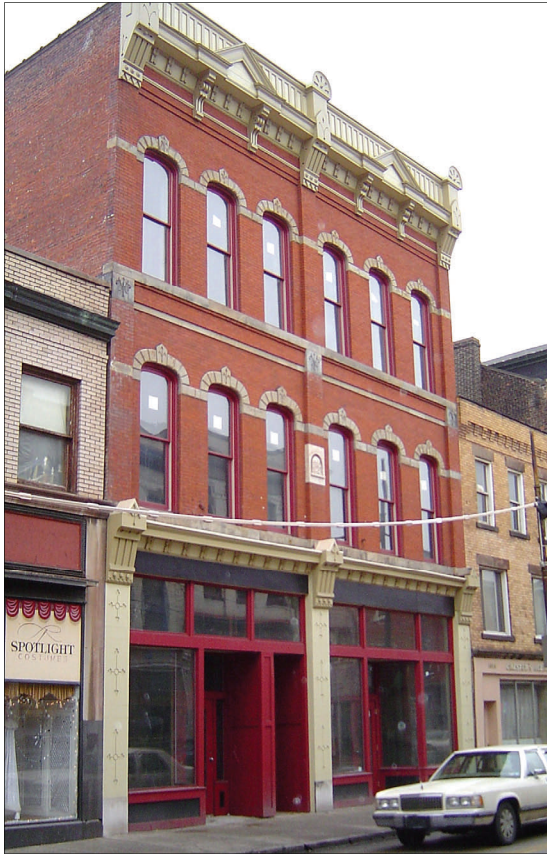
Figure 24. Brick façade cleaned and repointed
