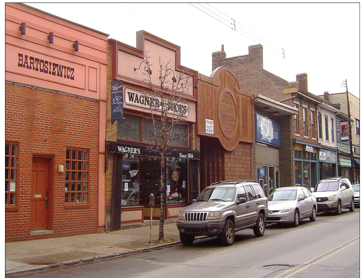
Figure 2. A mix of historic and remodeled storefront buildings
