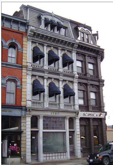
Figure 30. Awnings over window openings on upper floors
