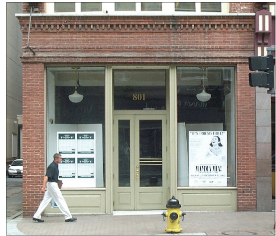
Figure 15. Glass storefront viewing zone
