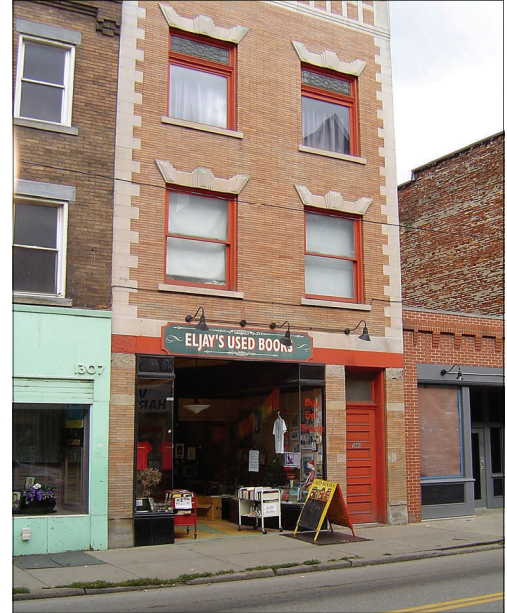
Figure 18. Intact storefront with paneled door to upper floors
